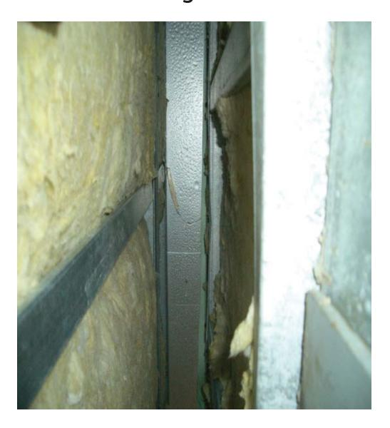
**Water droplets on cold framing.** When warm moist airleaks into in a wall cavity, it can hit the cool surface of framing, drywall, or exterior sheathing and condense. It is only a matter of time until it runs down the stud and becomes a puddle. Photo: EPA
