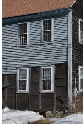
"A capillary break is either an air gap between adjacent layers or a material such as rubber sheeting that does not absorb or pass liquid water." — EPA
